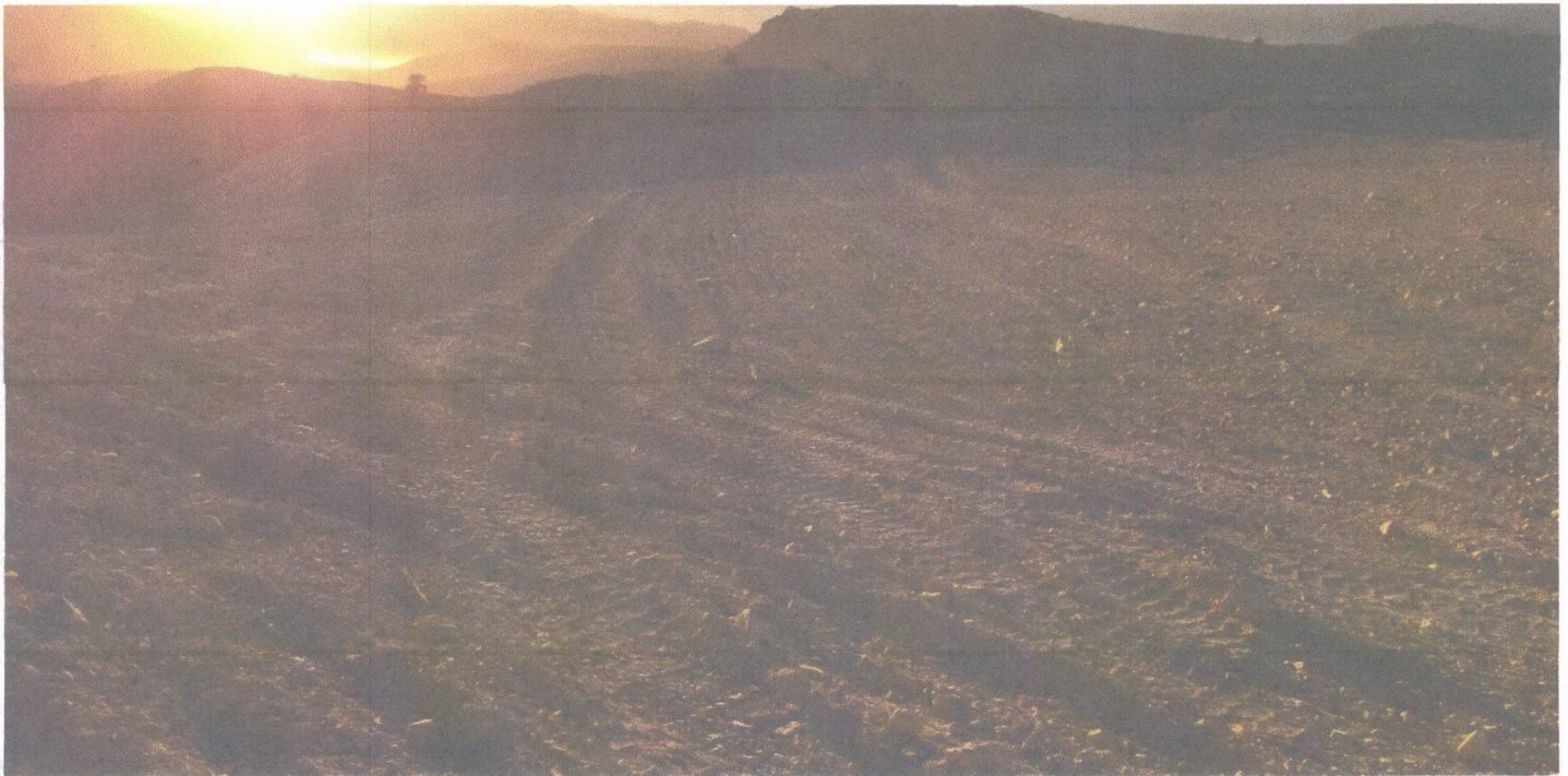
Photo 6: View facing west after top soil added and graded (December 2020)
