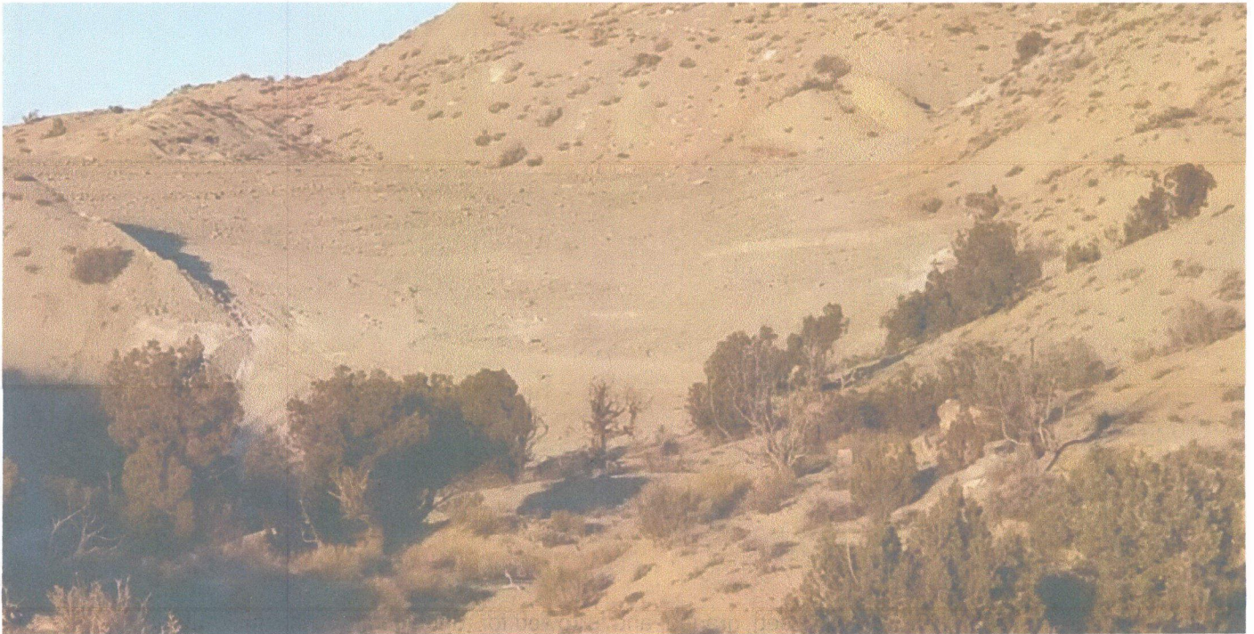
Photo 5: View facing north after top soil added and graded (December 2020)
